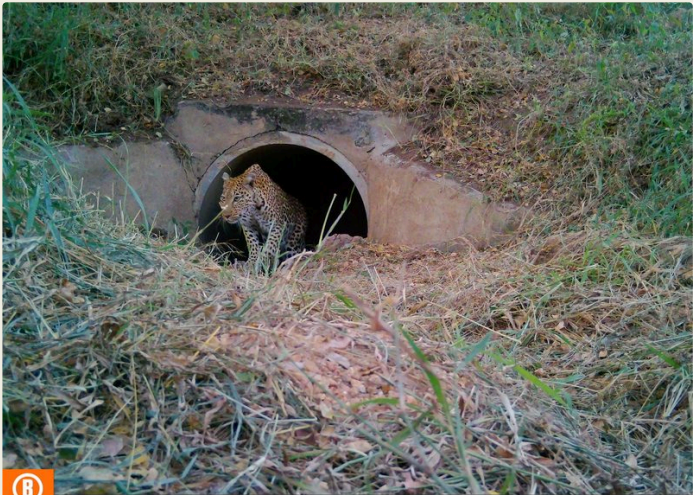
Bushnell CORE_CAM_33 68F 20C 06-11-2025 17:18:20 The Black Dot Female – camera trap, culvert survey
