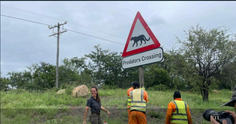
Installing signs with SANRAL on the R40
