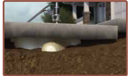
Poly foam is injected until void is filled or desired lift is achieved.
