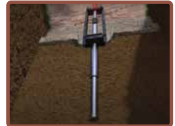
Pier sections are hydraulically driven to the point of refusal.
