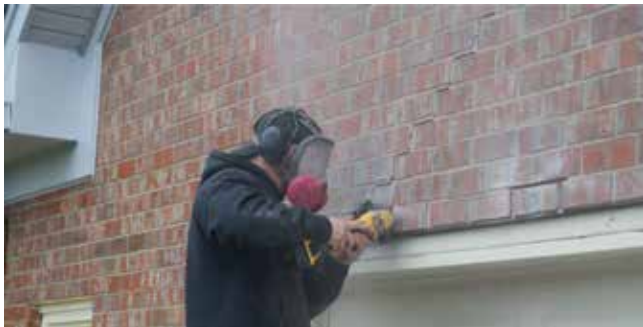
Bricks are carefully removed to access the lintel.
