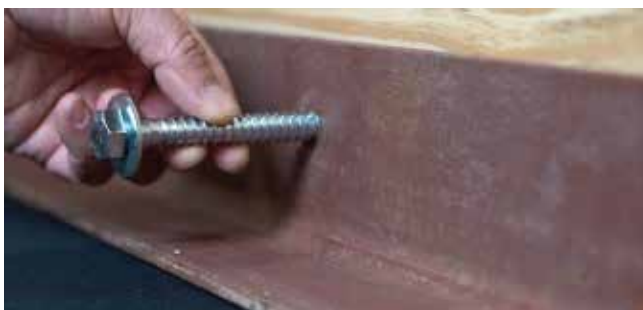
The lag bolts that are installed hold the lintel in place.
