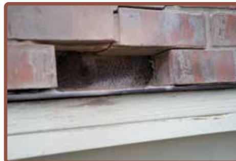
Removing the brick exposes the lintel. Rusted lintels must be replaced.
