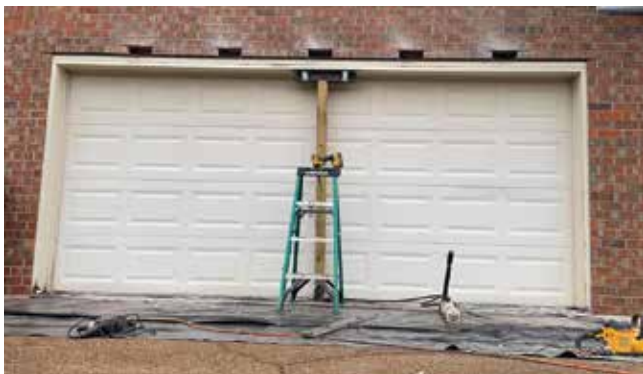
Additional support is provided during the lintel repair.
