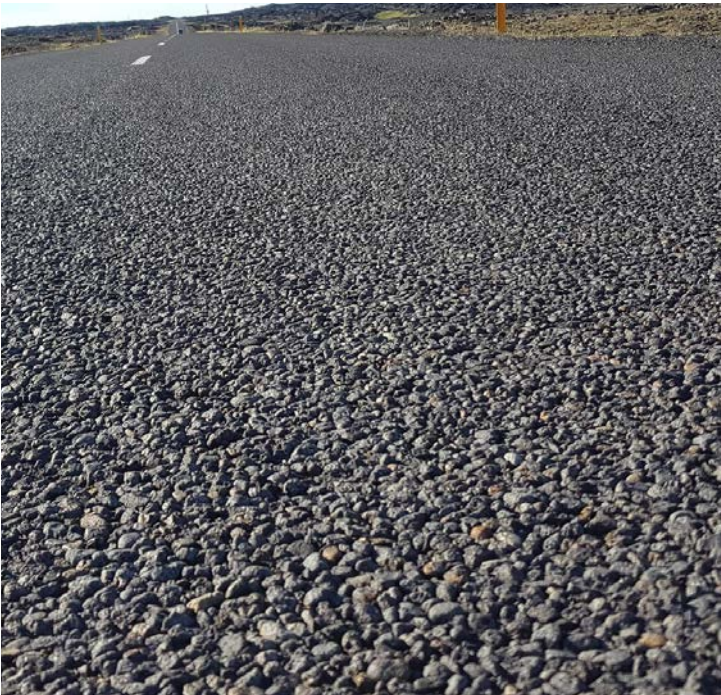
A Surface A - Chip seal concrete, to engineers specifications, for proposed site access in shared areas.
