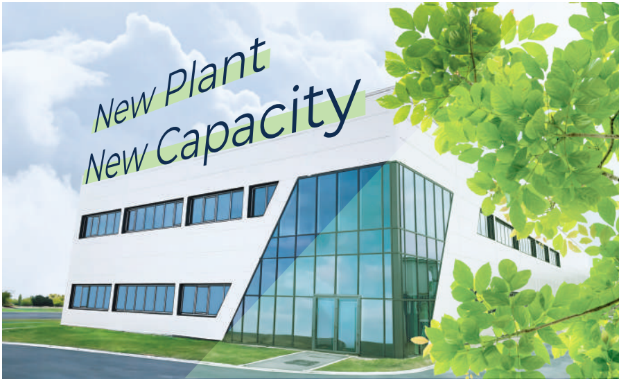
New plant, new capacity
