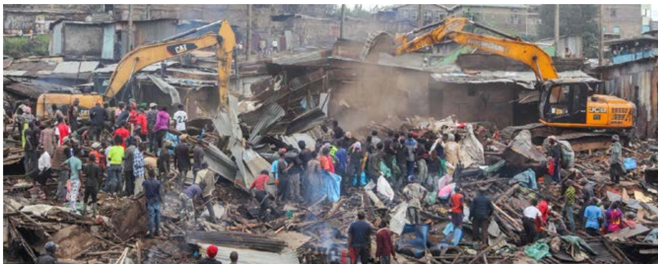
Bulldozers demolish homes along Nairobi's riparian zones in April 2024, as residents and Muungano members document the evictions to hold authorities accountable.
