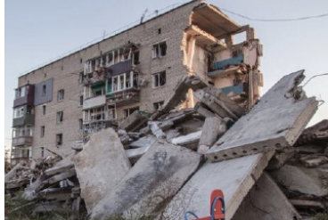
Concrete Reuse project - Ukraine © EPFL/Corentin Fivet
