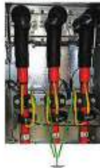
Fig. 3.3: Installation of three-phase sensor
