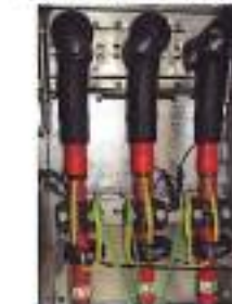
Fig. 3.3: Installation of current sensors
