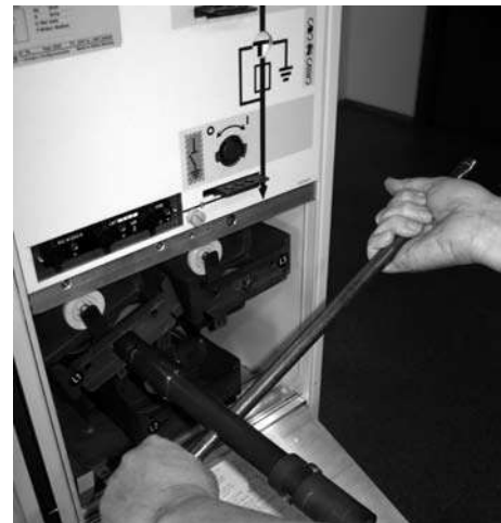
5. Applying the operating handle and turning anti-clockwise opens the fuse canisters.
