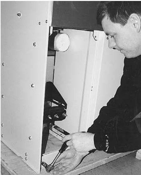
2. Removal of front section.
