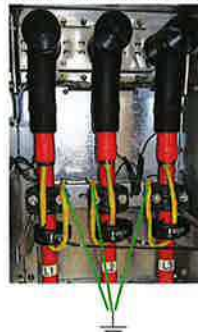
Fig. 3.3: Installation of current sensors
