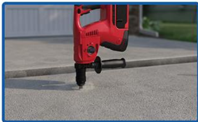
5/8" holes are drilled into the uneven concrete to allow for OxPoly ports.
