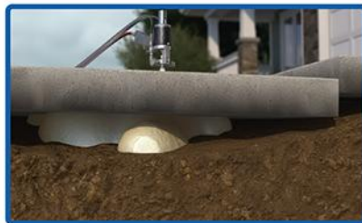
Poly foam is injected until void is filled or desired lift is achieved.
