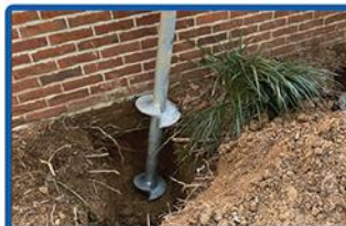
Area prepped with helical pier next to footer, ready for installation.
