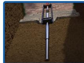
Push piers are hydraulically driven to the point of refusal.
