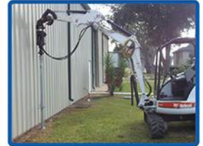
Equipment drives helical piers to the point of refusal.
