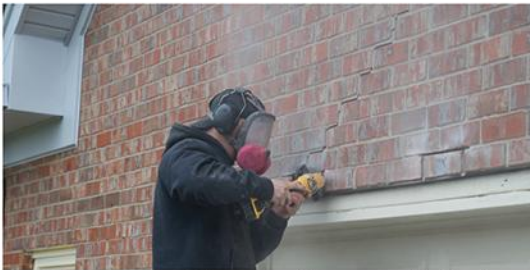
Bricks are carefully removed to access the lintel.
