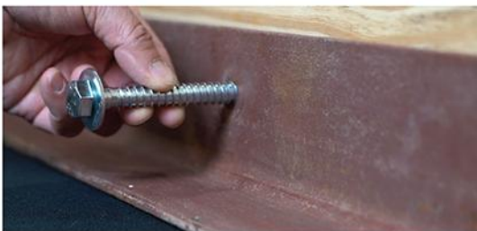
The lag bolts that are installed hold the lintel in place.
