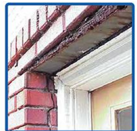
Removing the brick exposes the lintel. Rusted lintels must be replaced.
