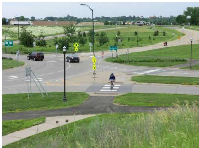
Example of a multi-lane roundabout.
