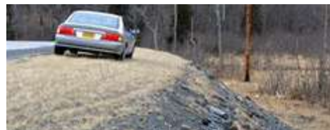
Shoulder is provided along roadway curve.
