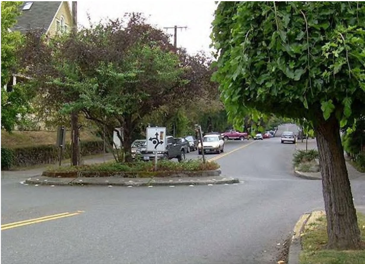
Figure 3.1. Horizontal Deflection Measure - Traffic Circle (Source: FHWA Module 1)
