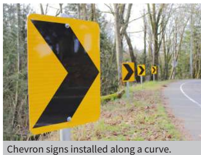
Chevron signs installed along a curve.
