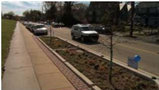
(Source: PennDOT Local Technical Assistance Program)
