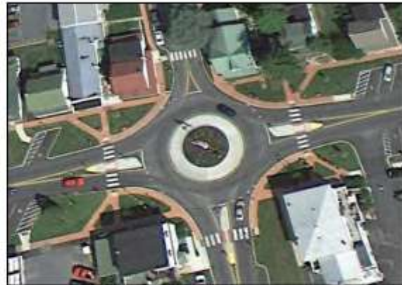
(Source: PennDOT Local Technical Assistance Program)
