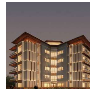
AKASA Davis Road Built up area: 27,000 sqft
