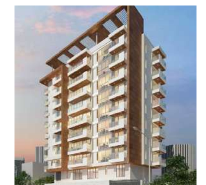
SKAV AHUJA LAGUNA Ulsoor Built up area: 35,000 sqft
