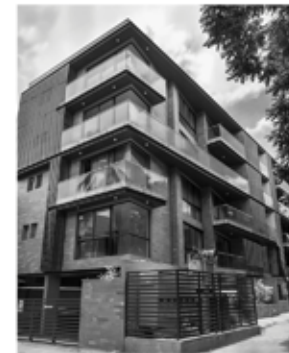
Residential SKAV Mehkri Ritz Cunningham Road
