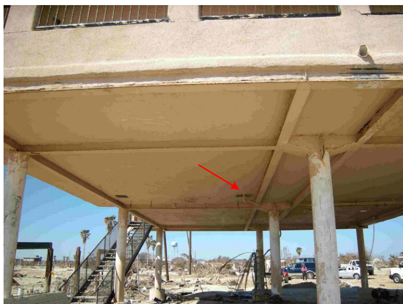
Figure 8.3-13. Photograph 3687. South elevation of house – Impact hole on underside of second floor deck, shown also in inset. The bottom hole was due to the concrete cracking when the railing was bent. (remove lower left arrow- drain)
