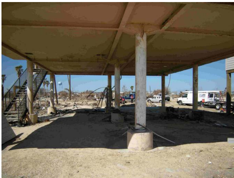
Figure 8.3-11. (101808d- 3688) View looking north under the house. Foundation of the Crystal Beach SCIP house did not sustain damage from Hurricane Ike.
