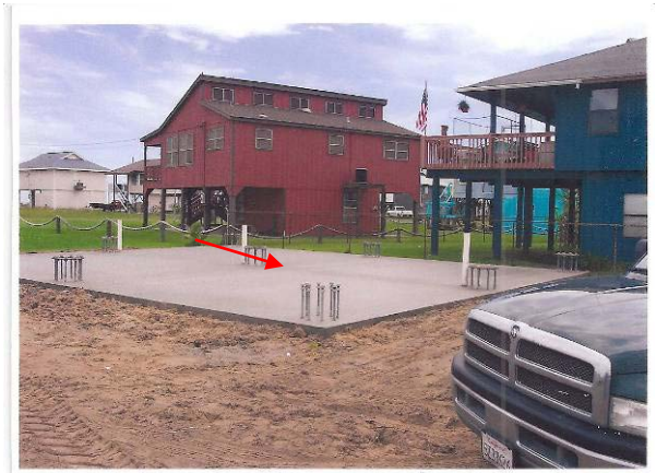
Figure 8.3-4. Construction photograph shows 24-inch deep bolts extending into the cement foundation (red arrow). The slab extends over the outside concrete foundation. Photo courtesy of Ron Bell.
