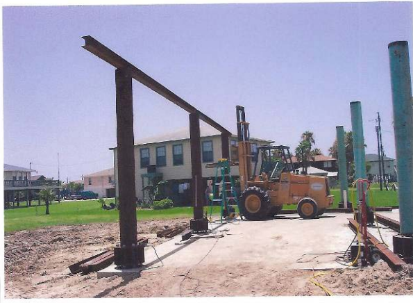
Figure 8.3-5. Construction photograph shows columns bolted in place. The nuts under the flange are used to level the 6-foot by 6-foot H beam. The rebar that will extend into the first floor vertical walls will be welded to the first floor (elevated) beam shown in the photograph. Photo courtesy of Ron Bell.
