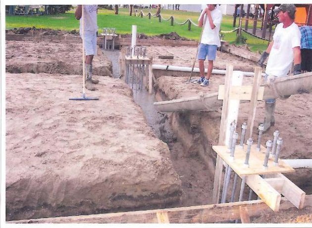
Figure 8.3-3. Construction photograph shows foundation with nine sets of bolts for the columns. There is a perimeter-grade beam and a center-grade beam. The men on the right are standing on sand at the height of the 6-inch slab. Photo courtesy of Ron Bell
