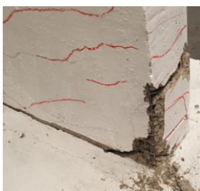
At failure (North)
