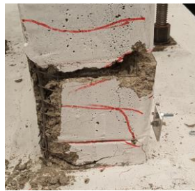
At failure (West)
