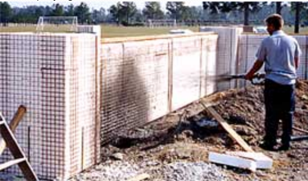
Spraying 3D Panels
