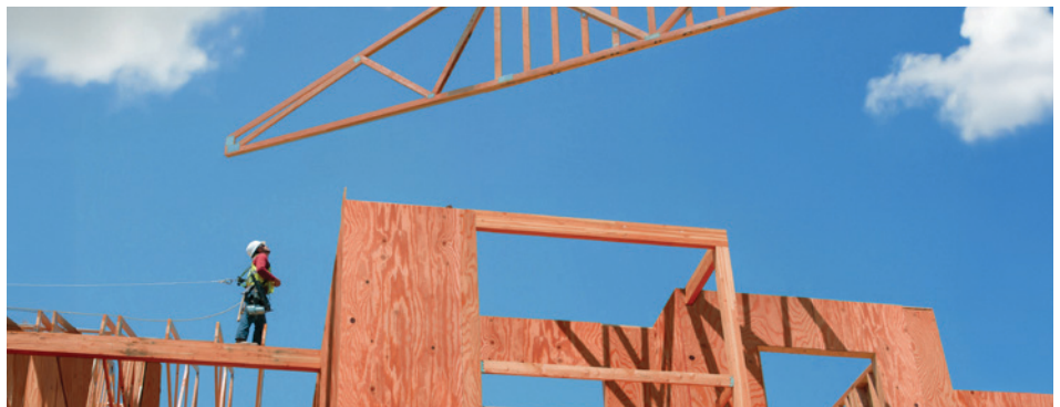
ProWood FR used in roofing systems can eliminate the need for sprinklers.
