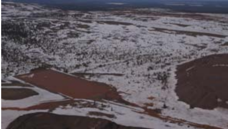
Figure 5. Aerial view of SP3 and associated infrastructure.
