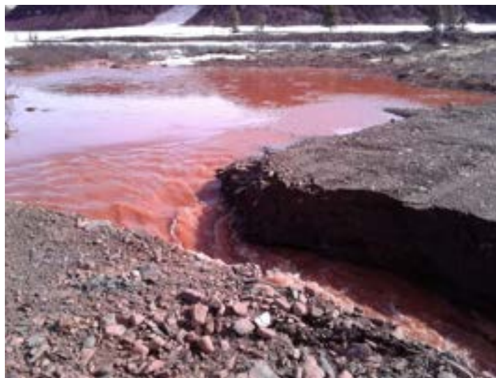
Figure 2. Closeup of breach at the SP3 SE corner, with water flowing into SP3.
