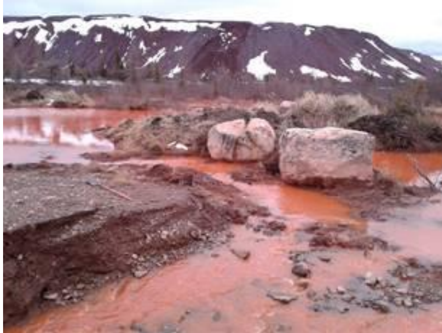
Figure 8. Inlet into breach, showing minimal water flow into SP3.
