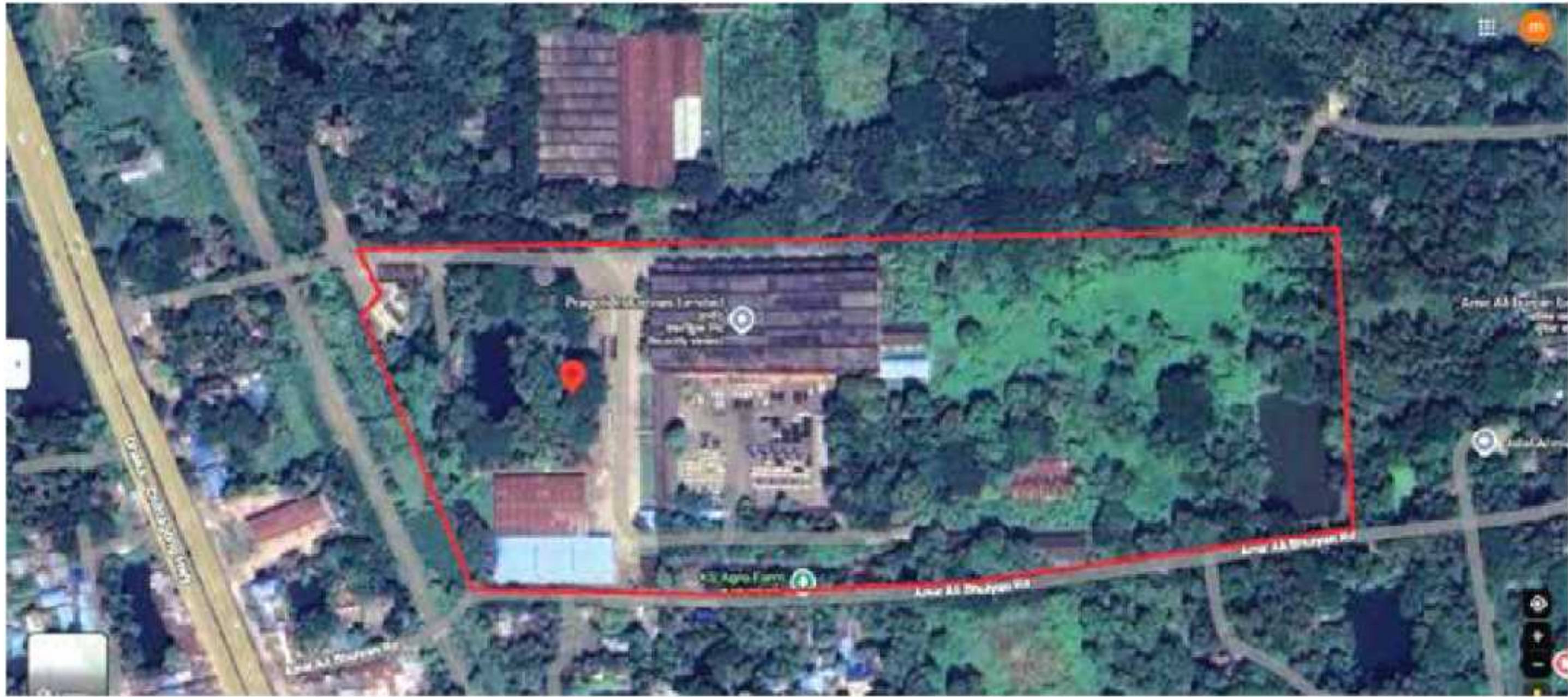
Aerial view of PIL, Nasirabad, Chattogram
