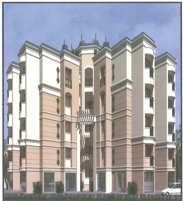
T.H. Road, Tondiarpet, Chennai - 600 081.
