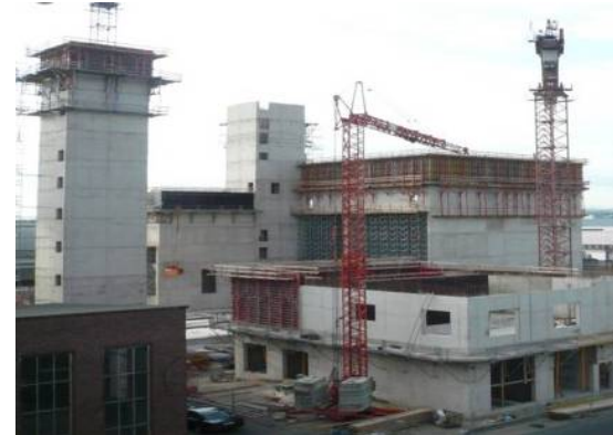
Andernach, Germany, 60 MWth, 65 t/a Sorted Waste – RDF
