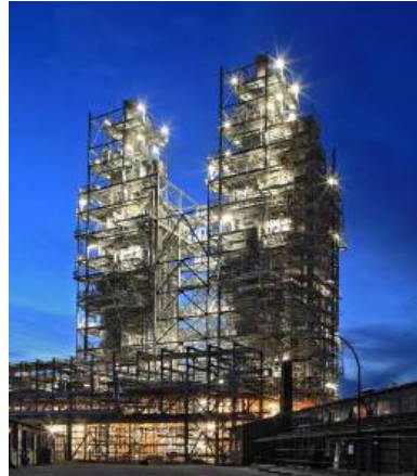
Dow Chemicals, Germany, 2 x 160 MWth Natural Gas and Hydrogen
