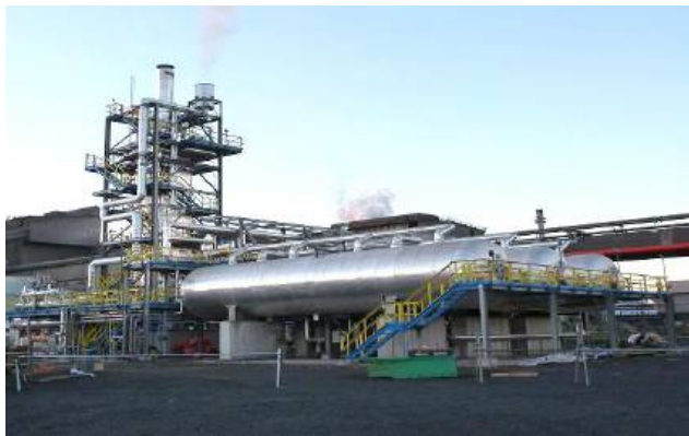
Tata Steel, Europe, 20 – 75 t/h Flue-Gas Quantity, 20.000 Nm 3 /h
