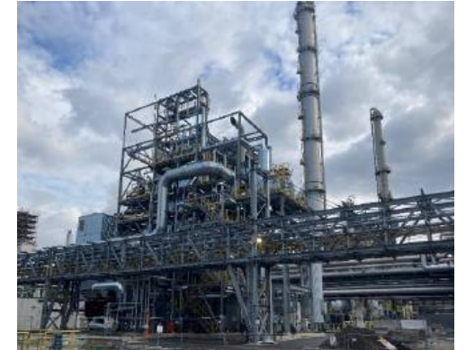
INEOS, Marl, Germany, 31 t/h, Liquid Waste
