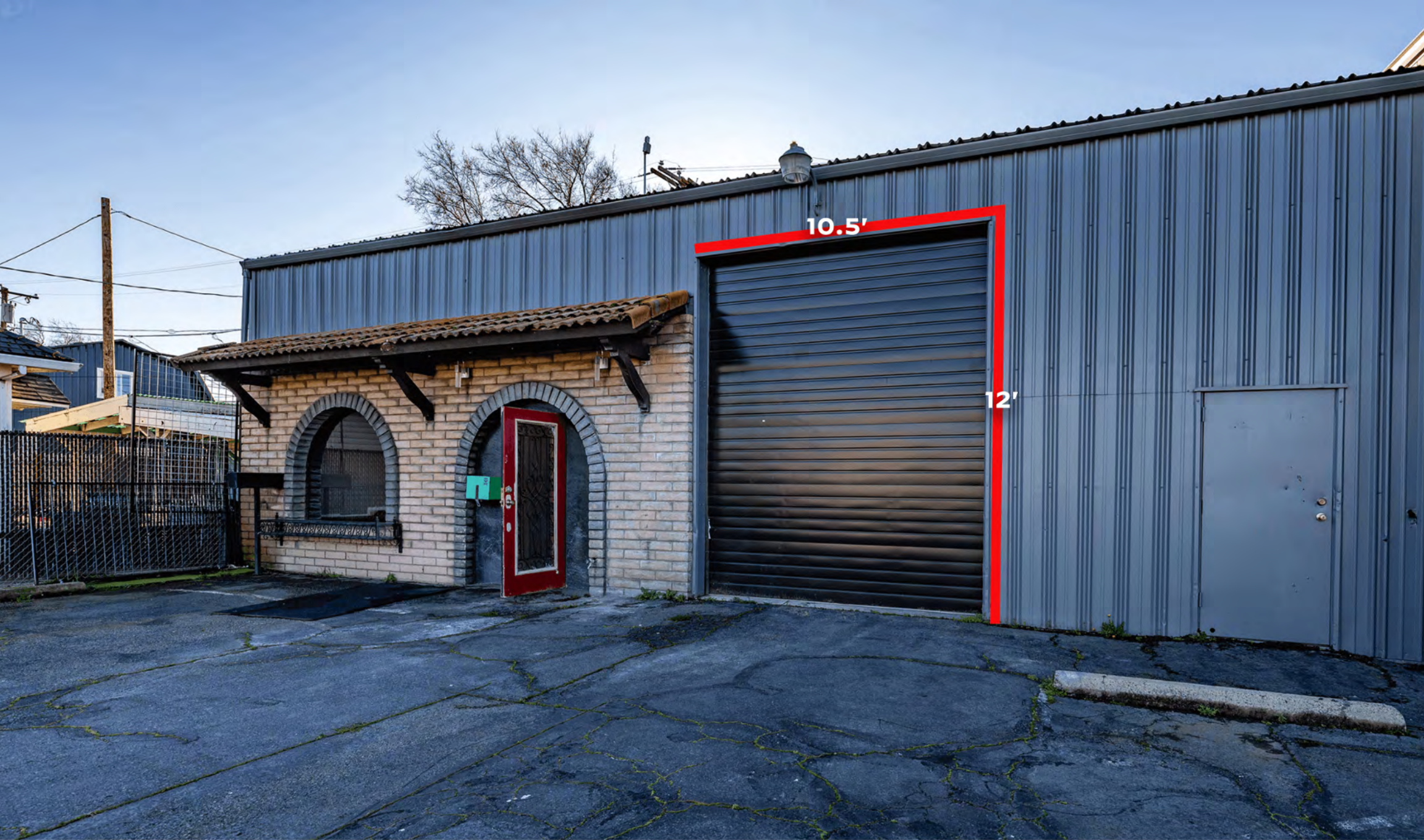
Subject Photo - Overhead Door
