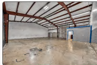
Warehouse 1 - SE View
