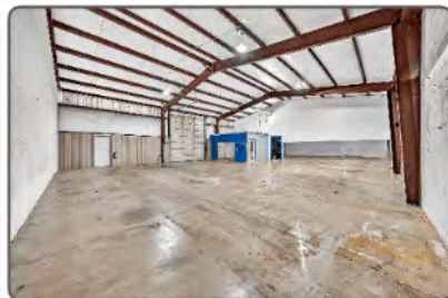
Warehouse 1 - SE View
