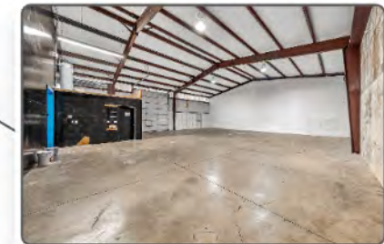
Warehouse 2 - SE View
