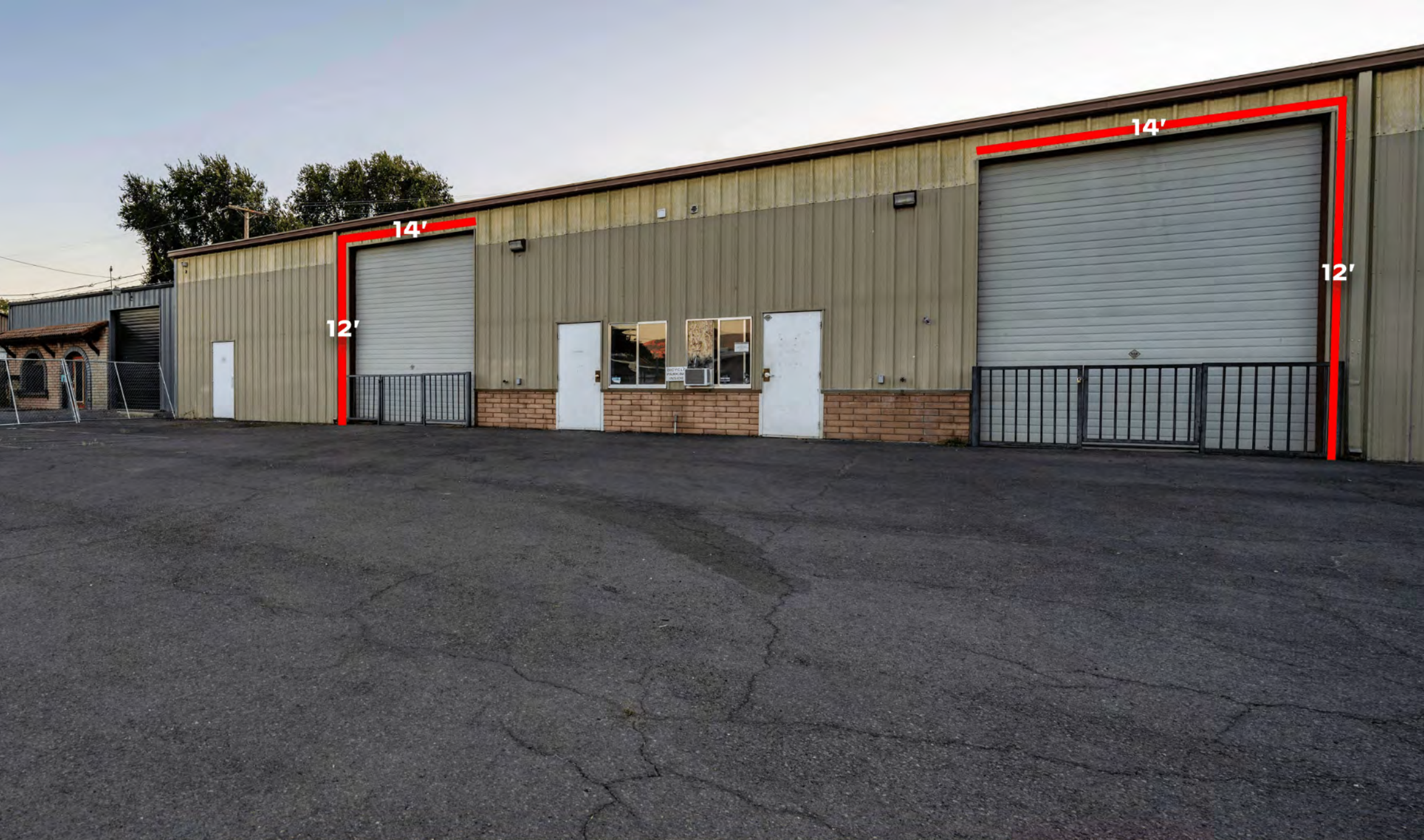
Subject Photo - Overhead Doors
