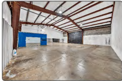
Warehouse 1 - SW View
