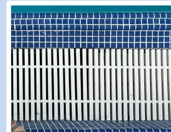
New pool basin surface
