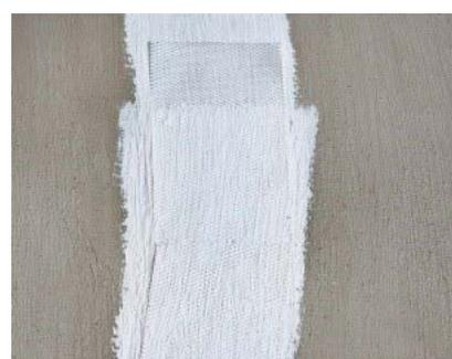
After cure, a final layer may be applied to smooth transitions and texture the repair. The whole area can be painted over with KÖSTER Renovation Paint White.
