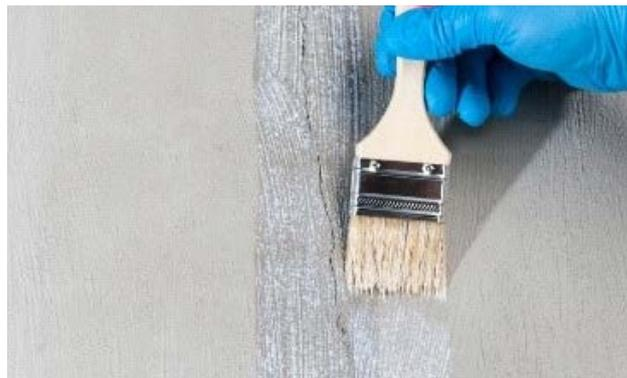
A layer of KÖSTER Dachflex (undiluted) is applied 15 cm wide over the crack. KÖSTER Flex Fabric is cut into 10 cm strips. The KÖSTER Flex fabric is embedded into the fresh material, overlapping the strips 5 cm. Immediately or after curing apply a second 20 cm wide layer of KÖSTER Dachflex over the KÖSTER Flex Fabric, so that the material is completely covered and the pattern of the KÖSTER Flex Fabric is no longer seen. The consumption per coat is approx. 130 - 175 g/m.
