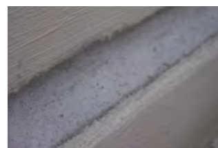
Round fillet made of KÖSTER WP Repair Mortar
