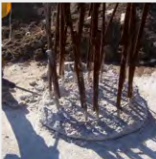
Removing protrusions, cleaning the pile head.
