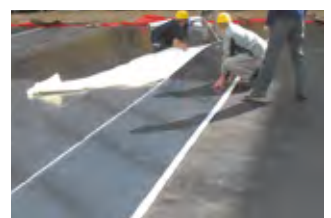
Waterproofing with KÖSTER KSK
