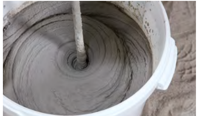
The powder component is slowly mixed into the liquid component in portions using an electric mixer. Mixing time is 3 minutes.
