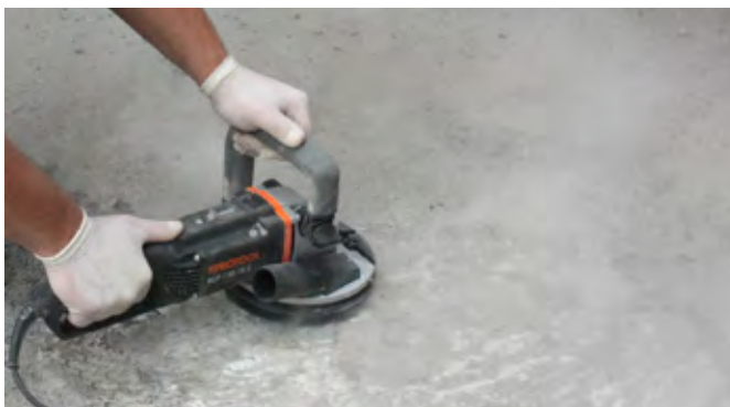
Substrate preparation
