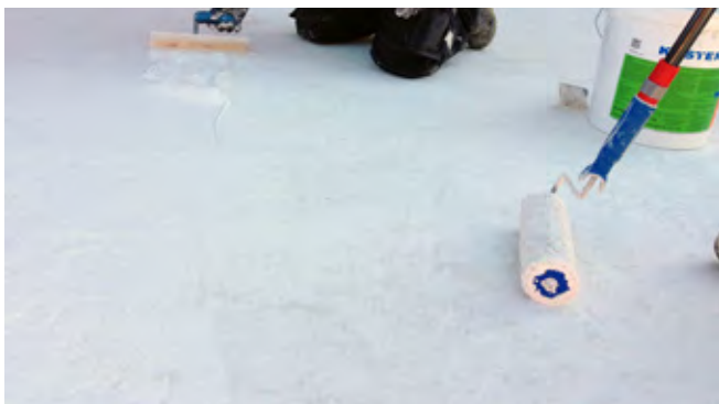
Application of the second layer of KÖSTER 21
