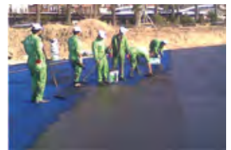
Waterproofing with KÖSTER Deuxan 2C
