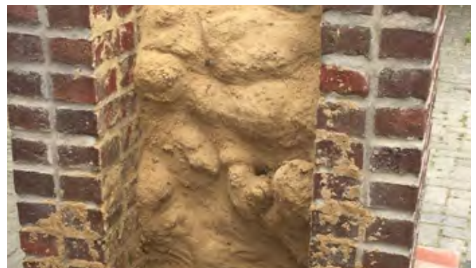
Curtain Injection (rear view)
