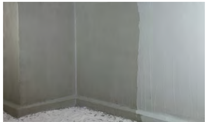
Application of the second layer of KÖSTER NB Elastic grey.
