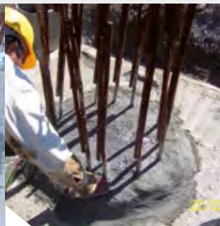
Waterproofing of the pile head with KÖSTER NB 1 Grey.
