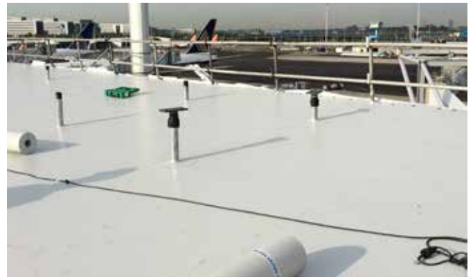
Flat roof waterproofing with KÖSTER TPO, Schiphol Airport, Amsterdam
