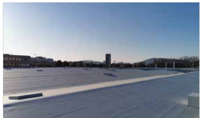
Roof waterproofing with KÖSTER TPO, Panama, Costa Del Este, food court, commercial property roof
