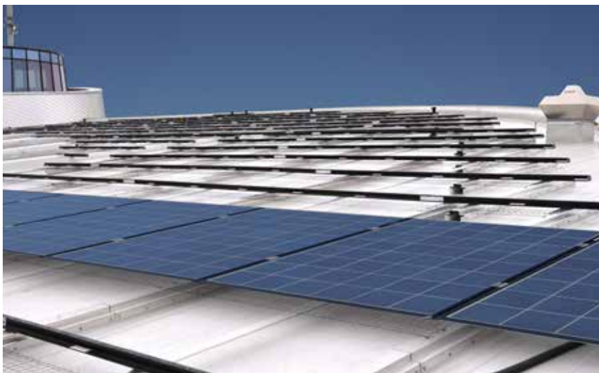
Mechanically fastened installation
