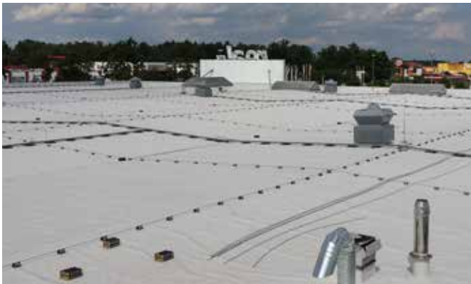
Flat roof waterproofing with KÖSTER TPO, REAL market in Gifhorn, Germany
