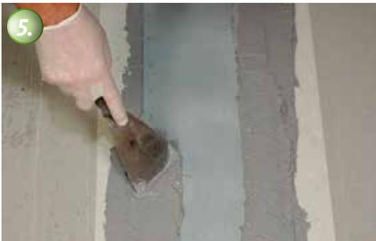
**5.** Immediately apply a second layer of adhesive on top of the tape and overlapping the masking tape on the sides. The center of the tape stays free of adhesive.
