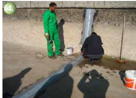
Connections are made with a hot air welding gun; seams should overlap at least 2 cm.
