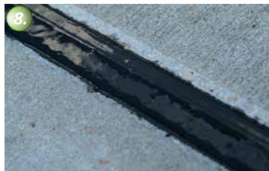
8. KÖSTER Joint Sealant FS-H in its cured state.
