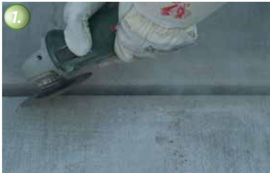
1. The joint flanks are beveled before the application of the Joint Sealant. The bevel must be at least 10 mm wide and in a 45° angle.
