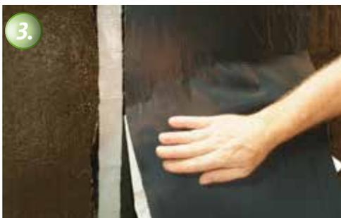
*Not only polymer modified bitumen thick film sealants, but also cold applied, self adhesive KÖSTER KSK Membranes are suitable for combining with KÖSTER Special Joint Tape for a reliable waterproofing.*
