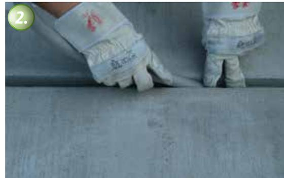
2. To avoid damages to the Joint Sealant caused by movement in multiple directions, the Joint Sealant should only bond to two joint flanks. For this reason a backing is installed for example with quartz sand or a foam PE backing rod. This eliminates the possibility of adhesion to three flanks.
