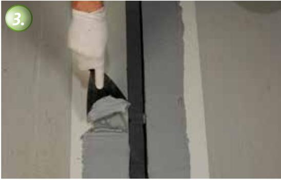
**3.** Mix the A and B components of KÖSTER KB-Pox Adhesive as stated in the technical guideline to a homogenous grey color. Apply KÖSTER KB-Pox Adhesive on both sides approx. 2 mm thick.
