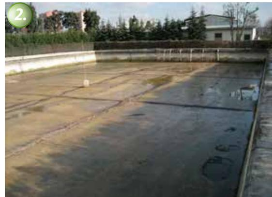
The surface is cleaned down to a solid and stable base material. The substrate must be clean, solid, and free from adhesion inhibiting materials.
