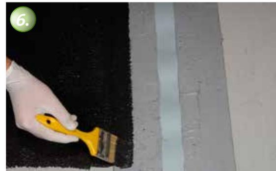
**6.** After KÖSTER KB-Pox Adhesive has cured for 24 hours, the area water-proofing can be applied overlapping onto the epoxy layer.
