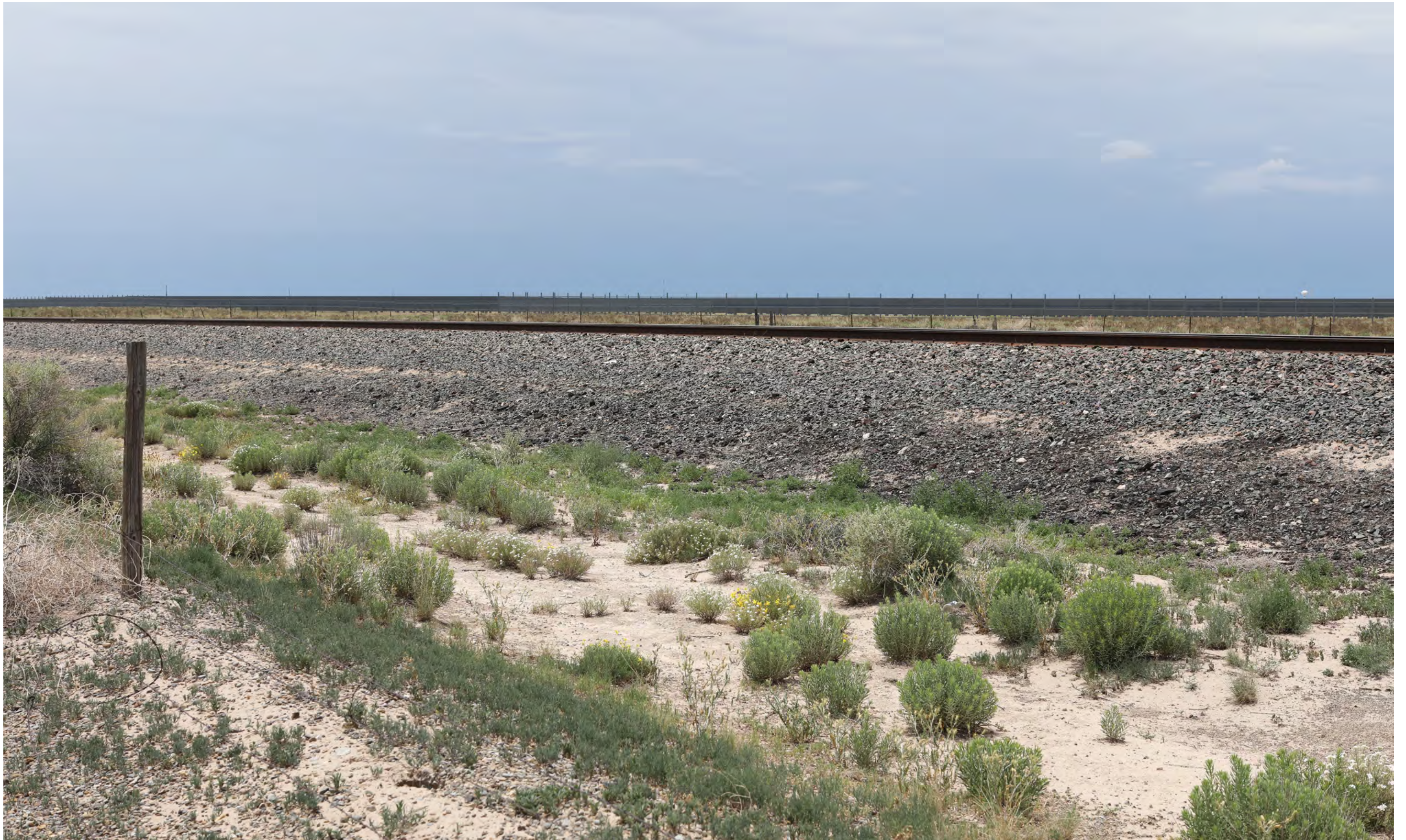
KOP 4: View from Wrangler Road looking west - Simulated Condition
