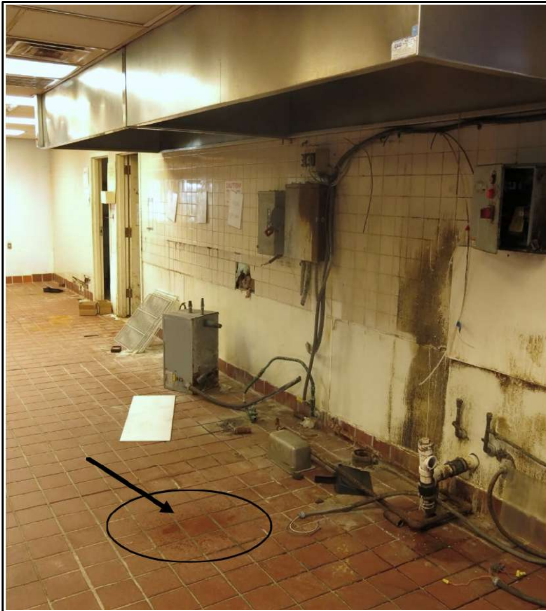
Figure 28. Leakage from ceiling piping or roofing.
