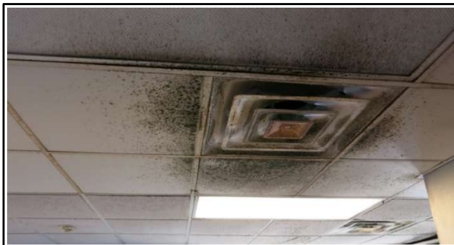
Figure 19. Mold growing near duct vents in Bldg. 2261.
