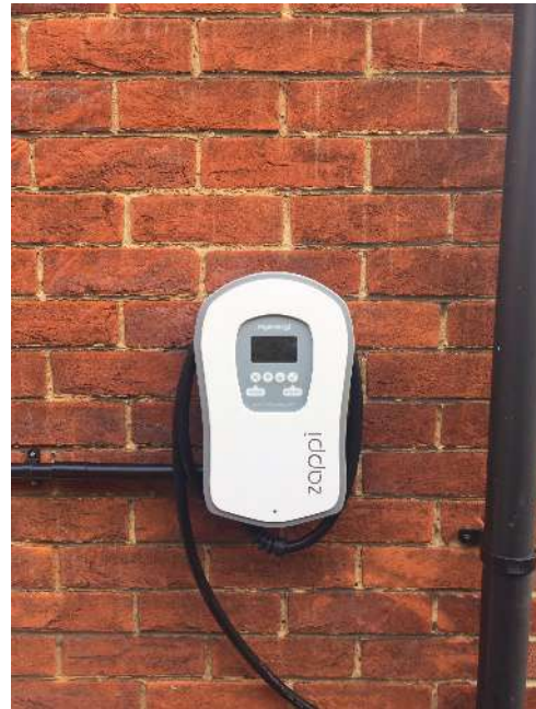
Figure 9: A wall-mounted EV chargepoint 16
