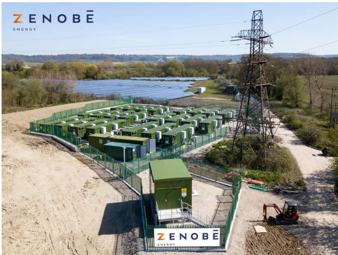
Figure 3: Zenobe's 29 MW battery storage site at Aylesford in Kent, co-located with a solar farm 8
