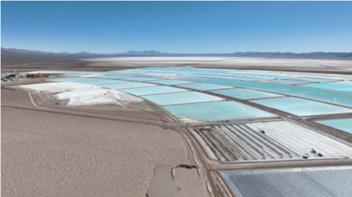
Figure 20.2 Olaroz Project – Evaporation Ponds and Facilities
