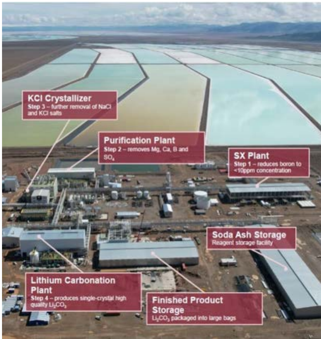
Figure 15.1 Aerial View - Main Facilities
