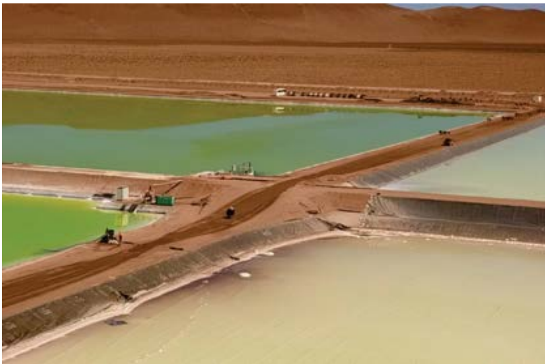
Figure 14.4 Evaporation Ponds – Close Up
