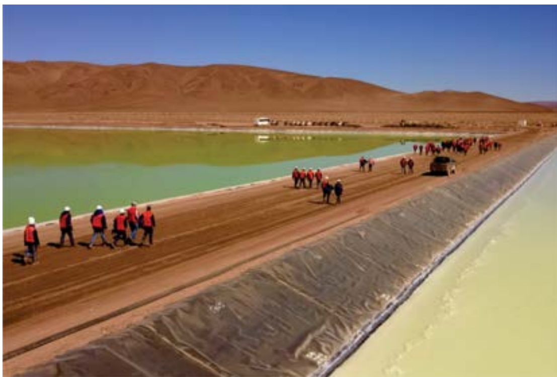
Figure 14.2 Evaporation Ponds at Cauchari Salar
