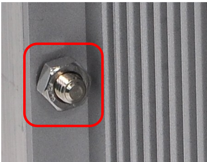
Ground screw of the switch
