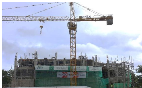
CBS Off-site Building
