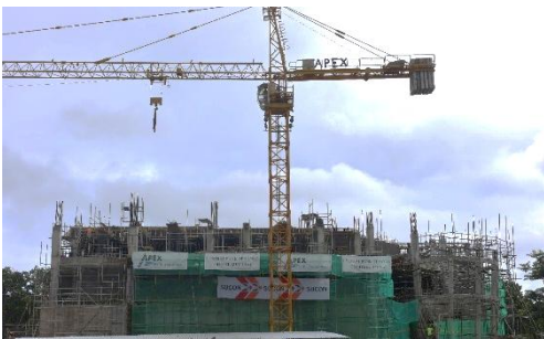
CBS Off-site Building
