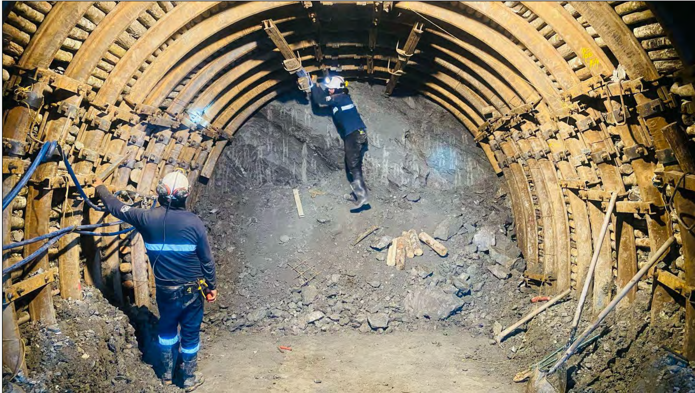
Underground decline development
