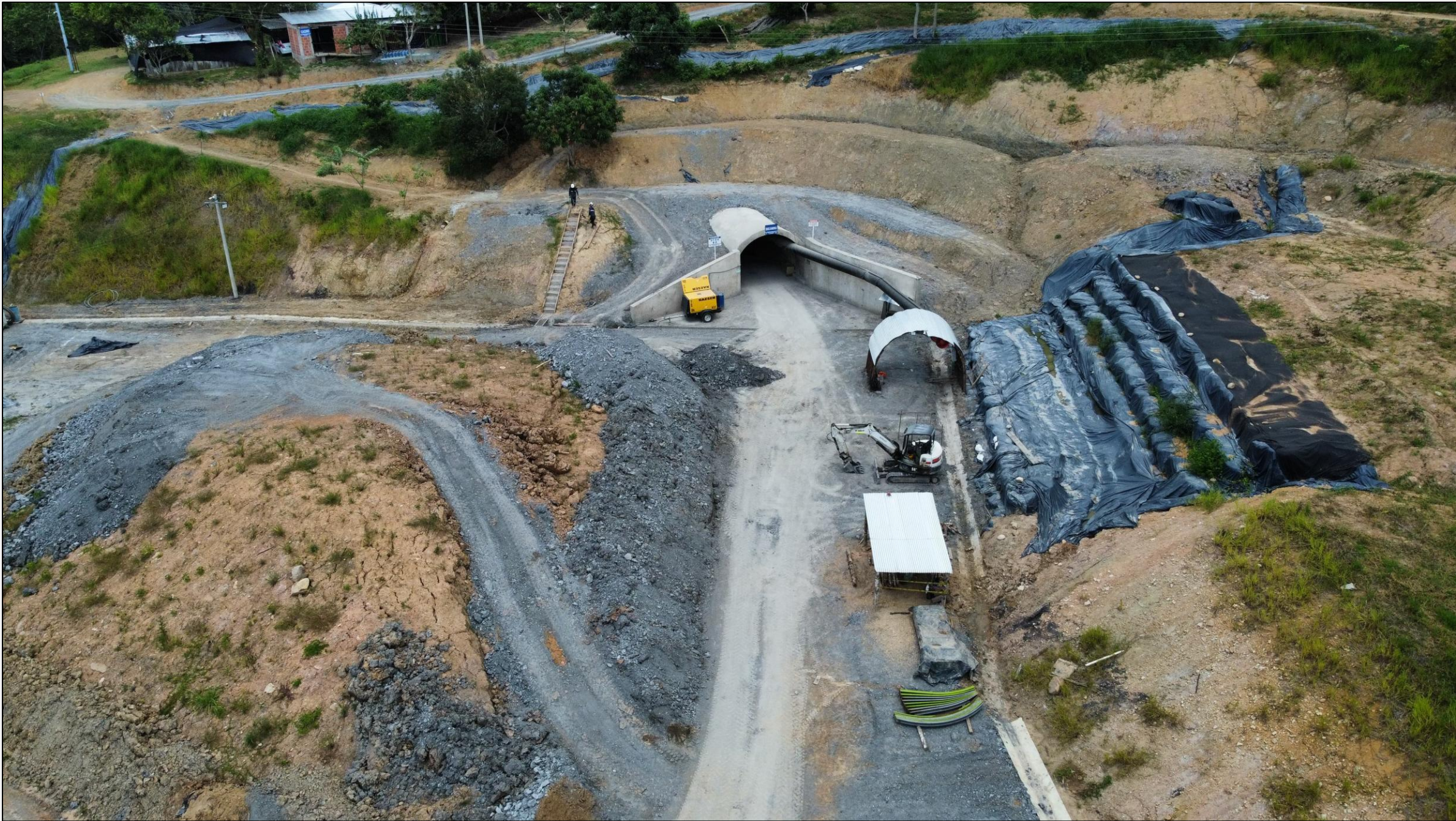
Portal Construction finalized March, 2025
