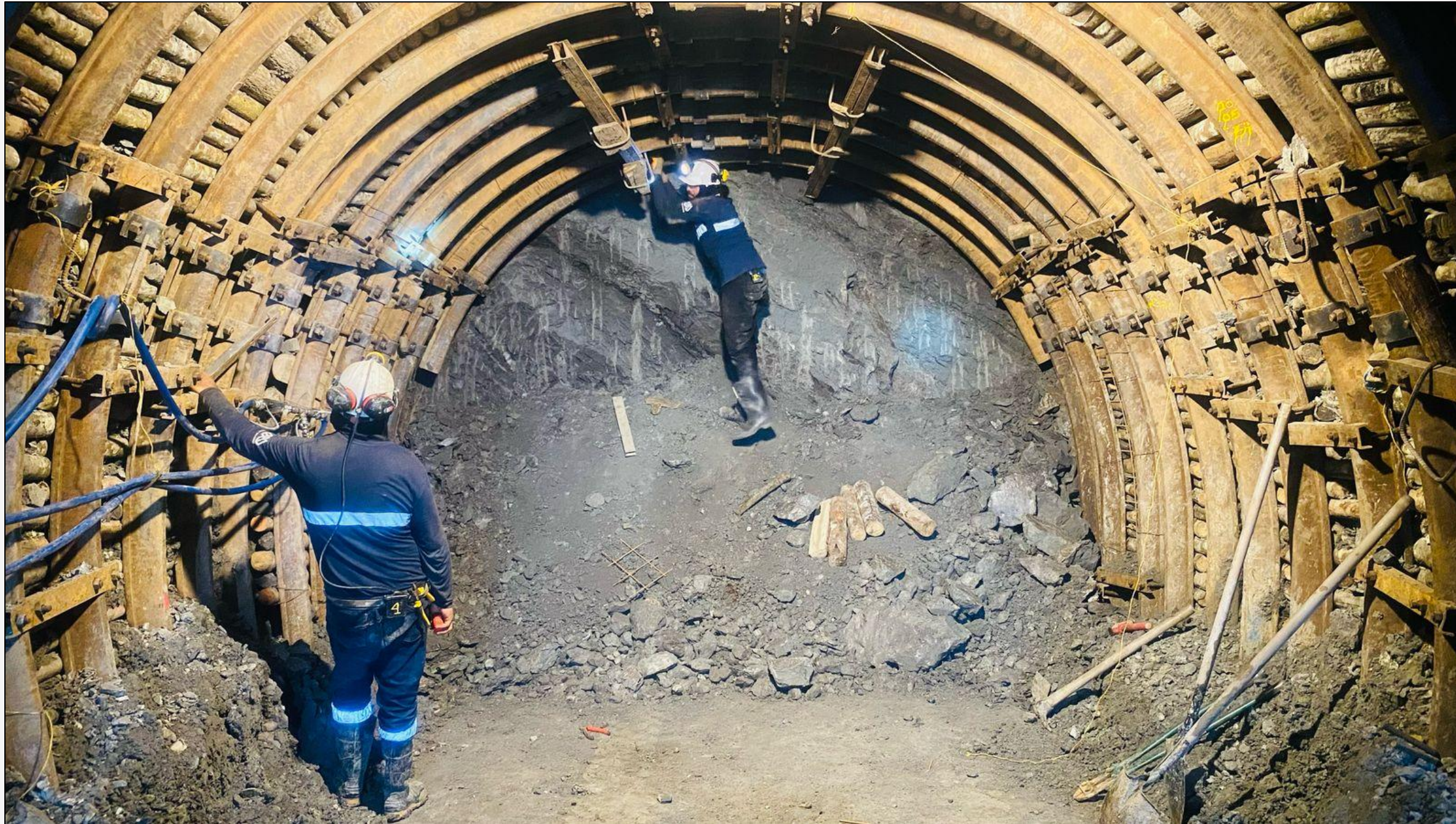
Underground decline development
