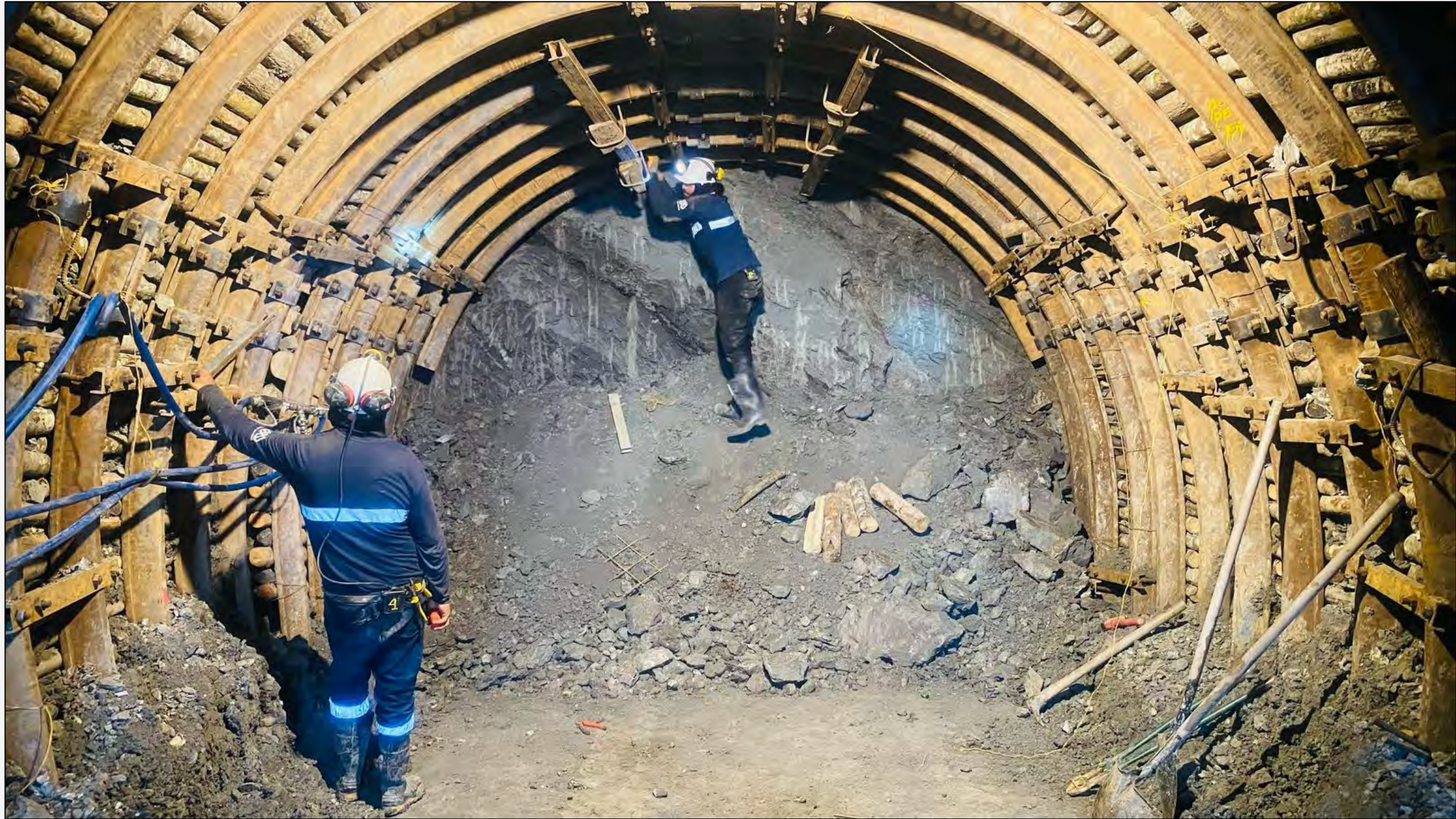
Underground decline development
