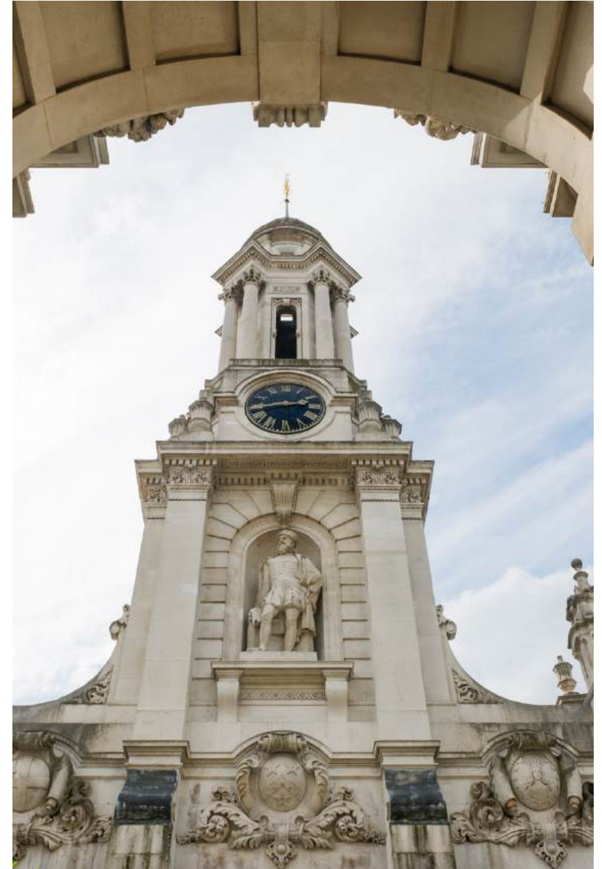
Contextual view from Second Floor terrace
