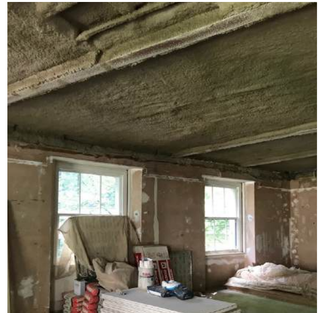
View following application of fire protection layer
