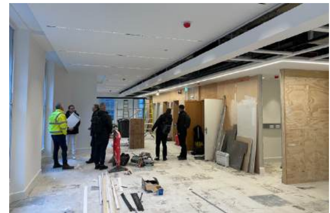
Sequential views of typical floor plate progressing towards completion.
