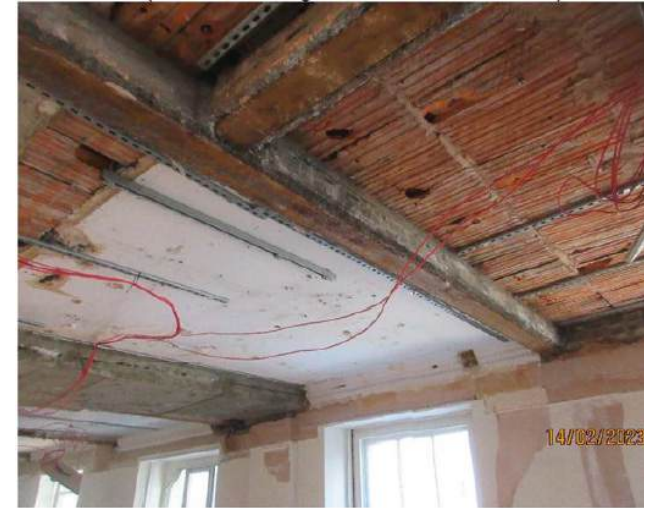
View of existing Farzzi floor system
