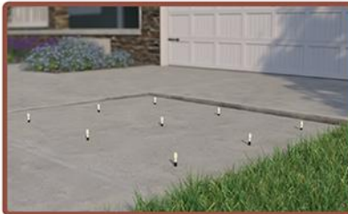
Ports are placed in drilled holes to inject two-part polyurethane foam.
