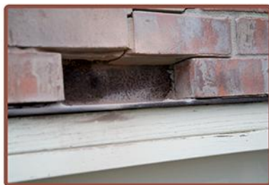
Removing the brick exposes the lintel. Rusted lintels must be replaced.
