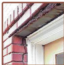
Removing the brick exposes the lintel. Rusted lintels must be replaced.
