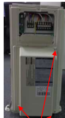
Screws of water collector
