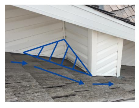
We will fix this by installing a slight slope behind your chimney to correctly direct water off of your roof.
