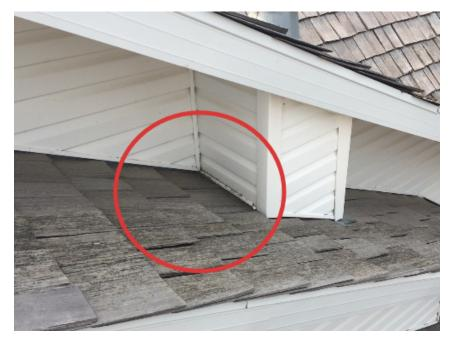
There is a "dead spot" behind your chimney. This is a low slope area that will allow water to pool on your roof, creating a very high risk of a leak.
