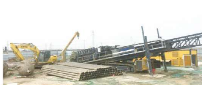
XZ13600, Oilpipeline, \Phi 1422\text{mm} , 700m
