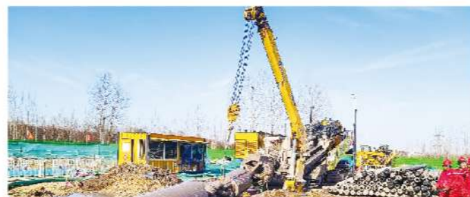
XZ11000, Natural gas pipeline, \Phi 1016\text{mm} , 2867m
